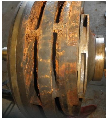
Figure 10: Original Diffuser Condition Side View
