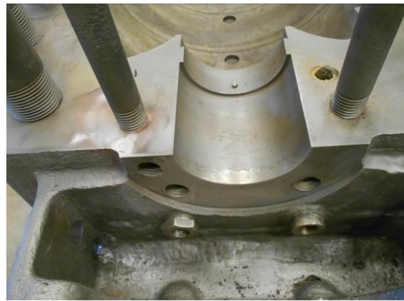
Figure 28: Water Jacket and Corners Repaired
